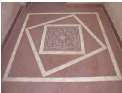
(Fig 42b): granite floor ,designed using the geometric movement: rotation, double interface , repetition of squares with common center and different dimensions.
